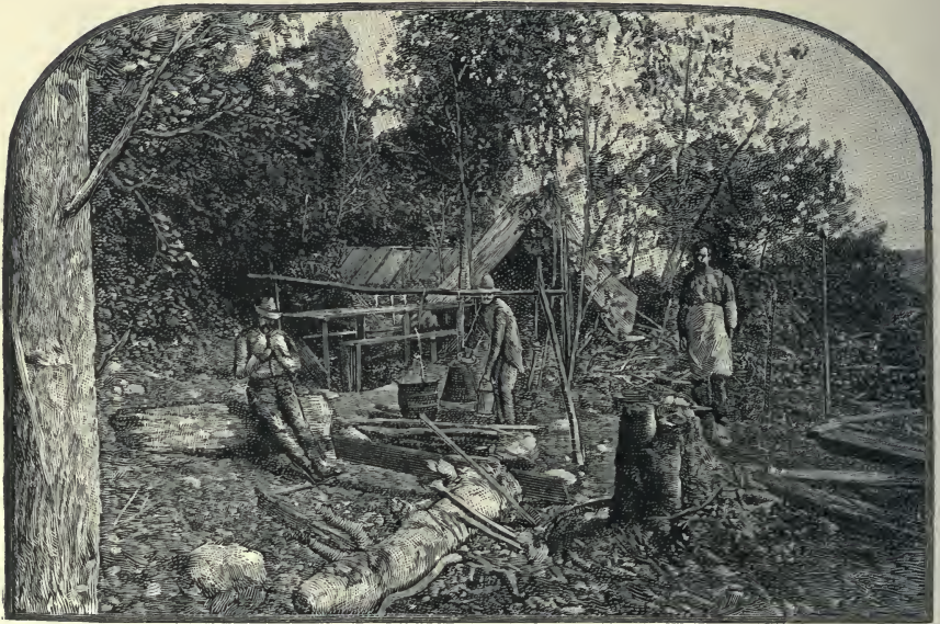
CAMPING OUT ON MIDDLE DAM CARRY.
